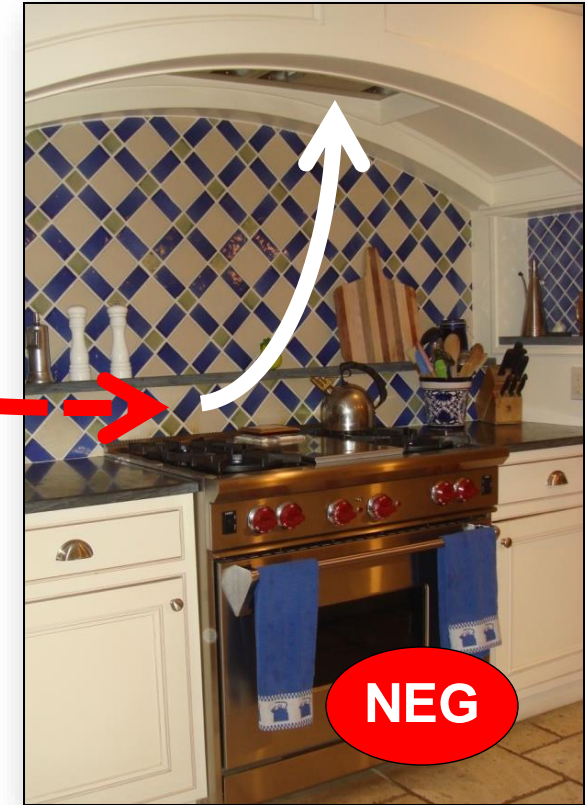
Caused by negative pressures in the kitchen
