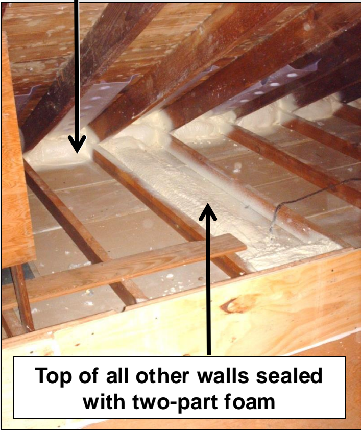
Top of outside walls and attic baffles foamed
